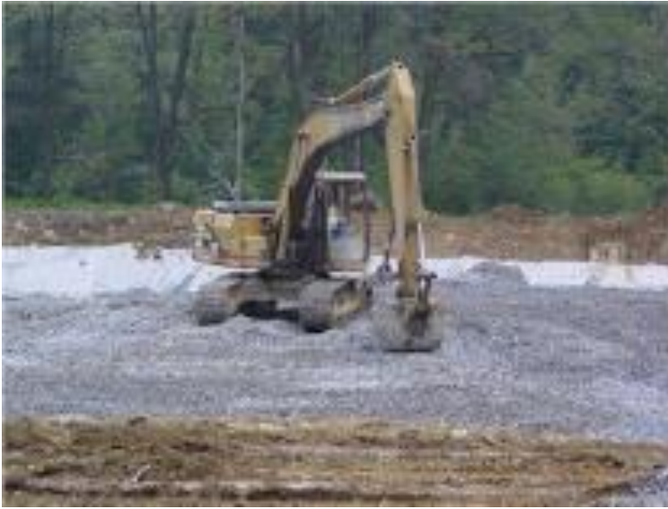
Figure 13: VFW Limestone Spreading (Hoover, K. L., & Rightnour, T. A. 2006)
