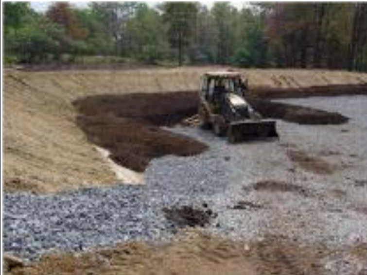
Figure 14: VFW Compost Spreading (Hoover, K. L., & Rightnour, T. A. 2006)
