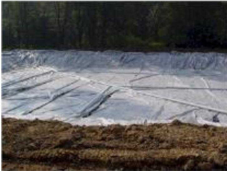
Figure 12: VFW Underdrain and Liner (Hoover, K. L., & Rightnour, T. A. 2006)
